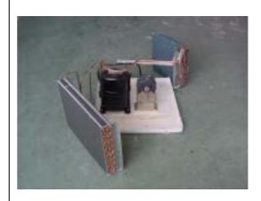
(16)Removal of fan motor assembly
